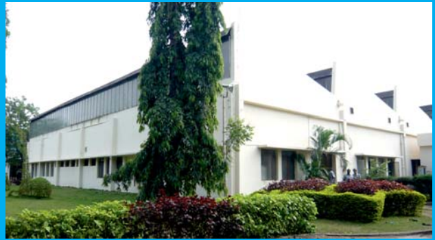
Hydraulic Pumps & Motors Plant
