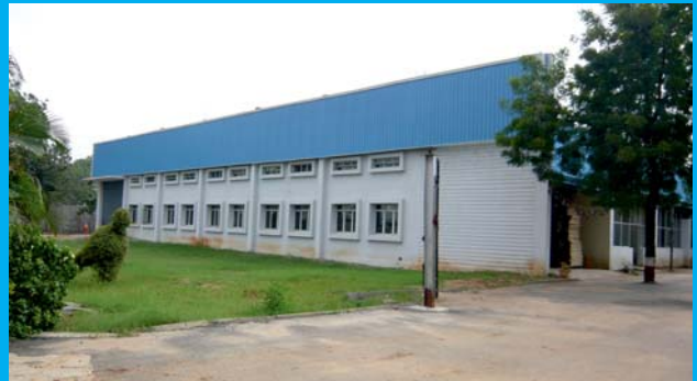
Hydraulic Valves Plant
